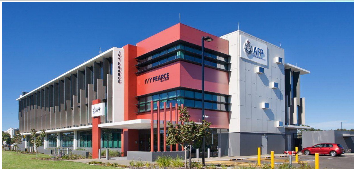
AUSTRALIAN FEDERAL POLICE BUILDING Australia – Brisbane 2016 5 units
